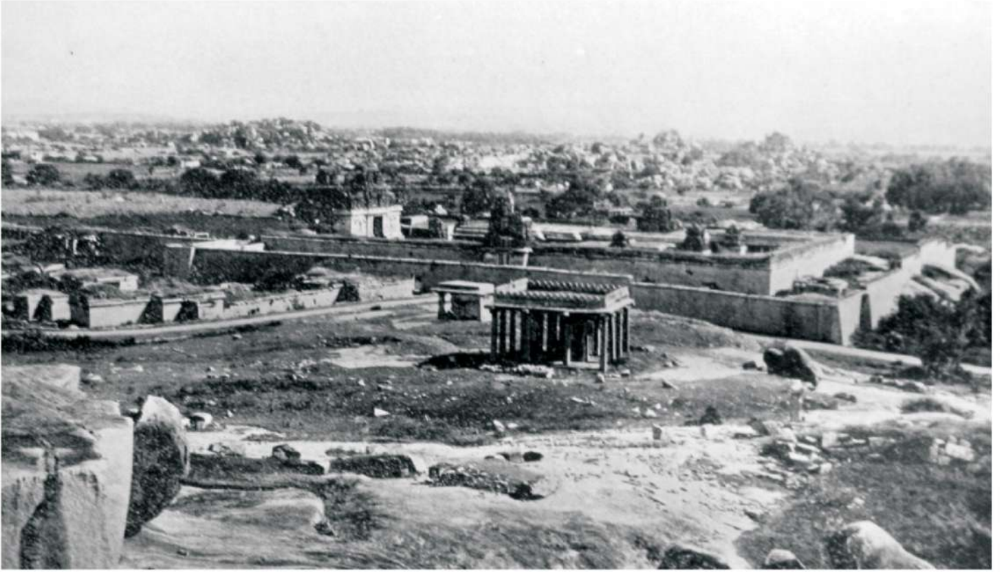
Fig.1A : Kṛṣṇāpura before renovation (Archaeological Survey of India, Southern circle report)
