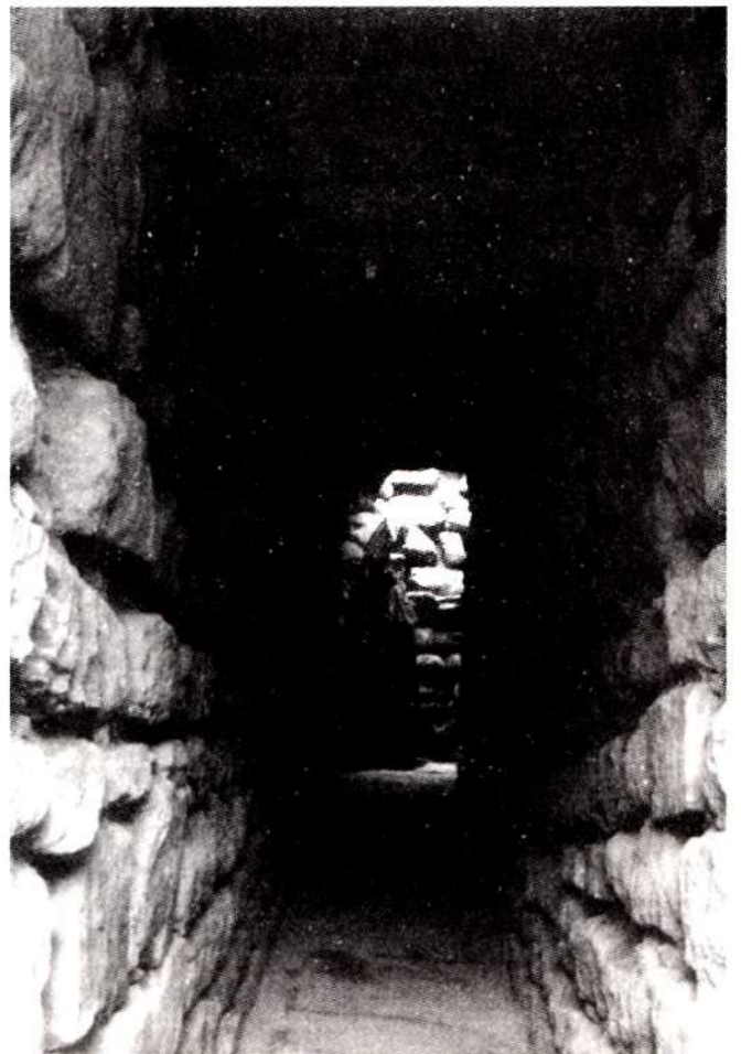
Fig. 6 : Inside of storm water drain in castle
