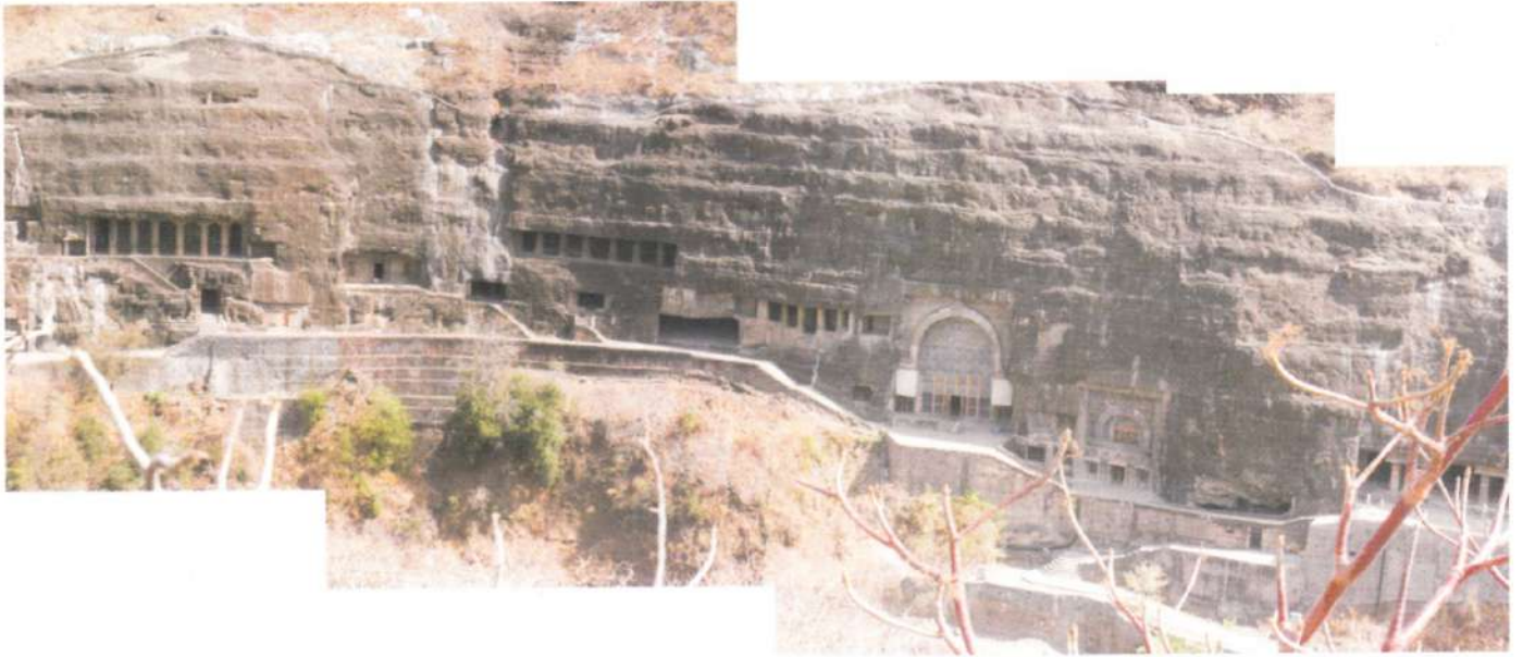
10.3: General View of Ajanta - Caves 7-16
