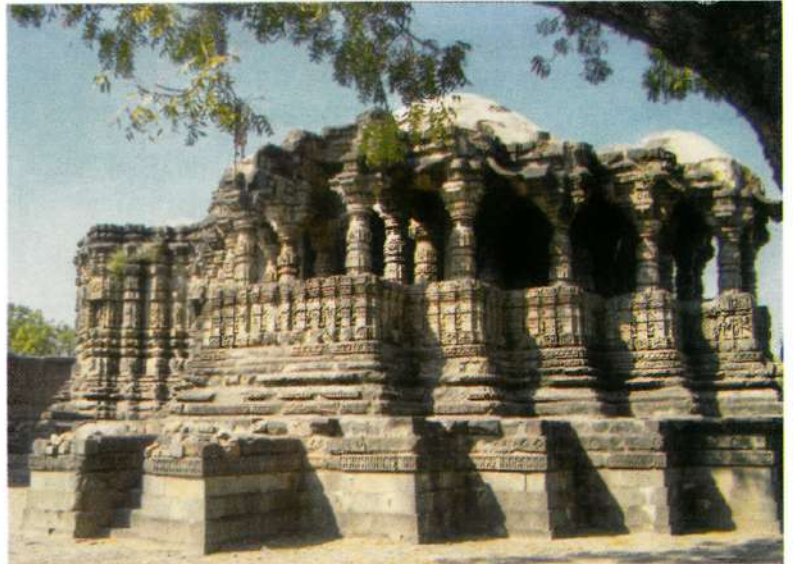
Fig. 1 : View from south-east, Anwā
